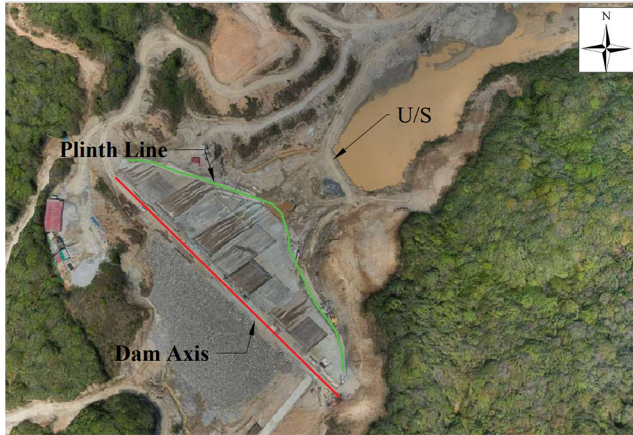
Figure 1.2: Drone Image of Under Construction Dhap CFRD
