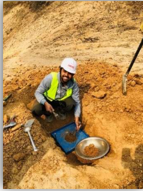
Figure 1: Field Density Test
