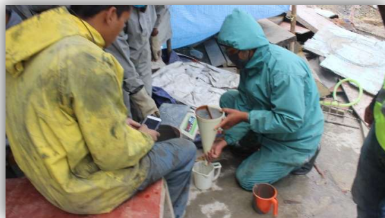
Figure 15: Flow cone test on grouting
