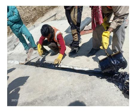
Fig: Bitumen pouring inside chamfered portion of joint
