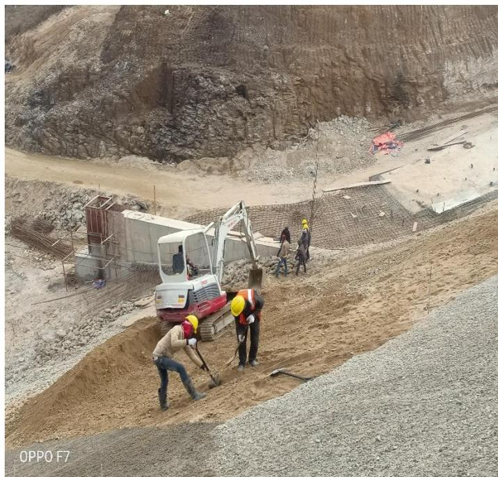
Fig: Removing 2B zone material near permanent outlet where slope is flatter than design slope.
