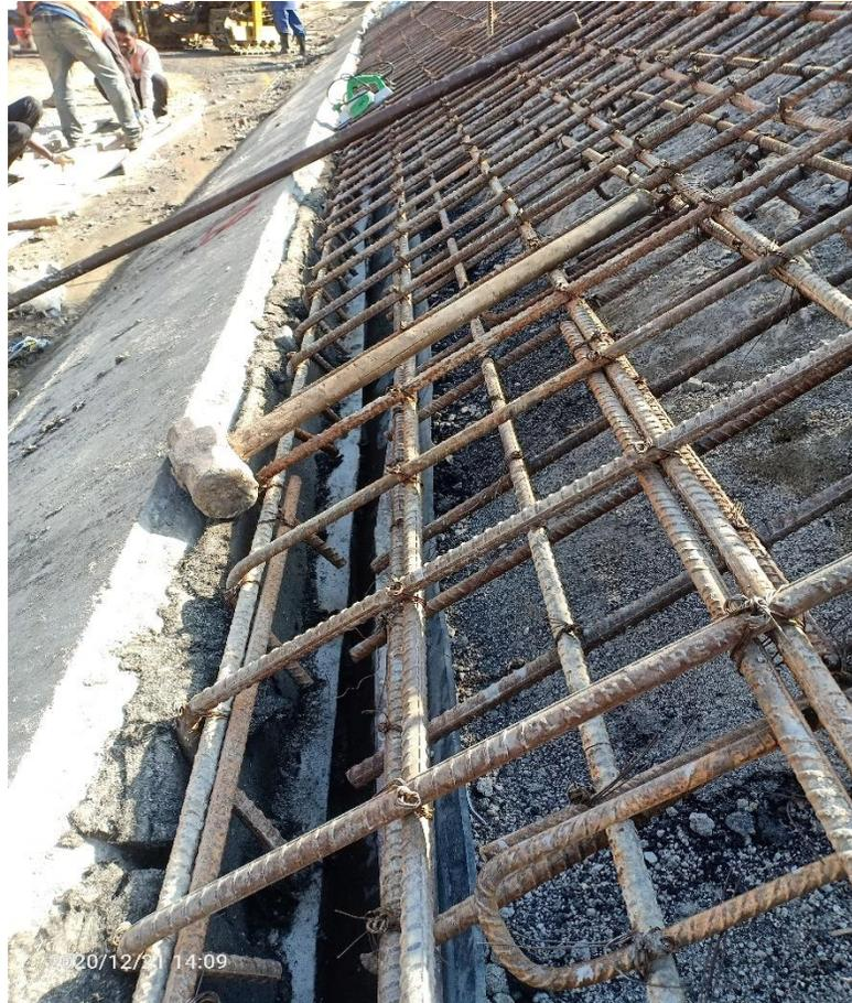
Fig: Damaging of bituminous fiber during laying of reinforcement bars.
