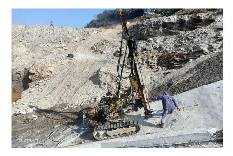
Fig: Normal drilling with ROC macchine
