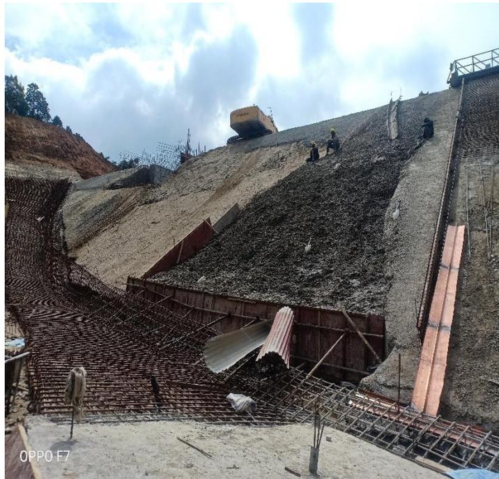
Fig: Pouring corrective lean concrete at S-10 panel as slope correction
