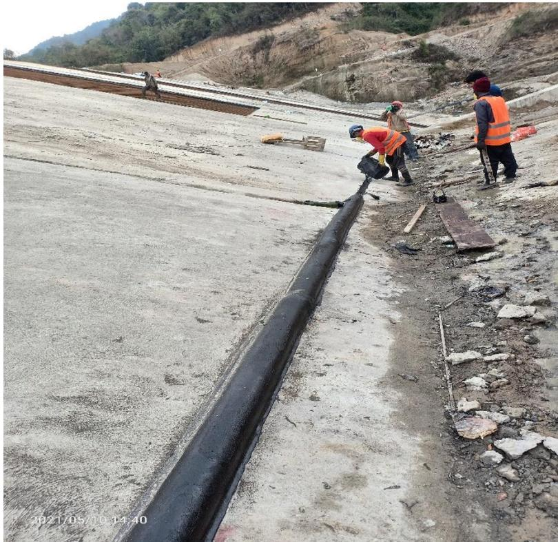
Fig: Final shape of the mastic mound at perimeter joint
