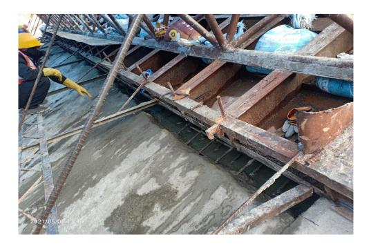
Fig: No overlap of slipform within starter slab. Chances of concrete leaking from this gap is high.
