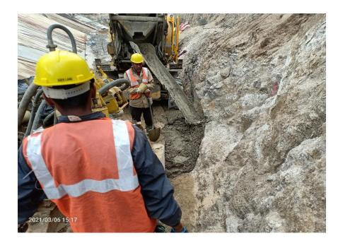
Fig: Lean concreting in trench adjacent to external plinth to minimize grout leakages.
