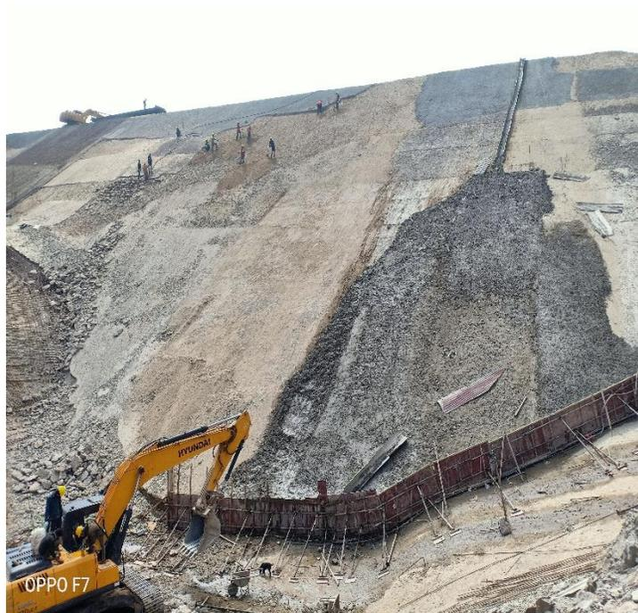
Fig: Slope correction by scrapping 2B material above permanent outlet and adding lean concrete on the surface near deepest section.
