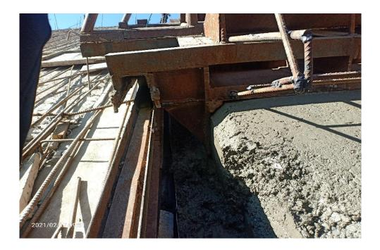
Fig: Moving side plate of slipform not able to hold the concrete and concrete is covering whole rib portion of the copper water stopper which necessitates manual chamfering.
