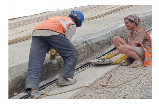
Fig: Repairing honeycomb concrete with repairing mortar
