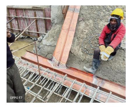
Fig: Joint at intersection of vertical and horizontal copper water stopper
