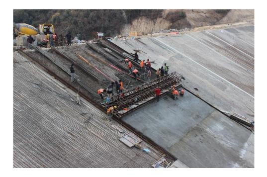
Fig: Concrete casting of S-9 panel using slipform
