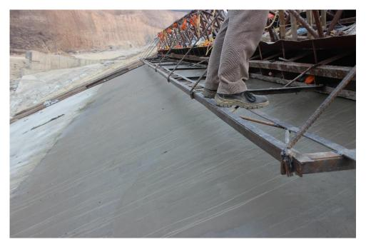
Fig: Finished surface of face slab
