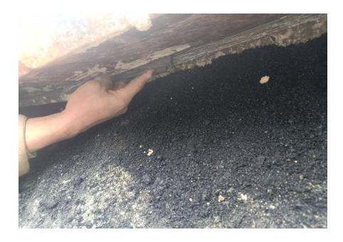
Fig: Filling the gap along the length of neoprene at joints.
