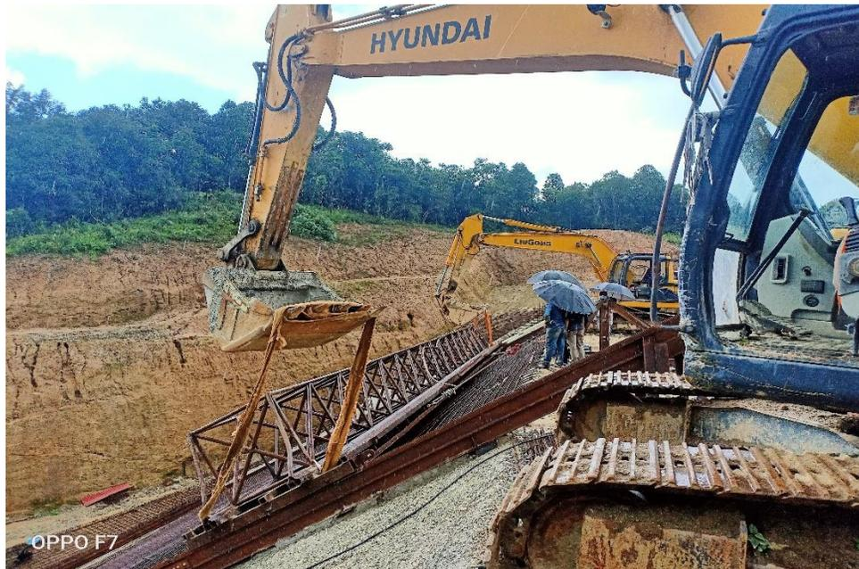
Fig: Loading Slipform on rail for trial running
