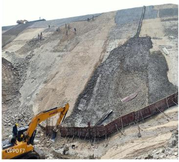
Fig: Slope correction by scrapping 2B material above permanent outlet and adding lean concrete on the surface near deepest section.
