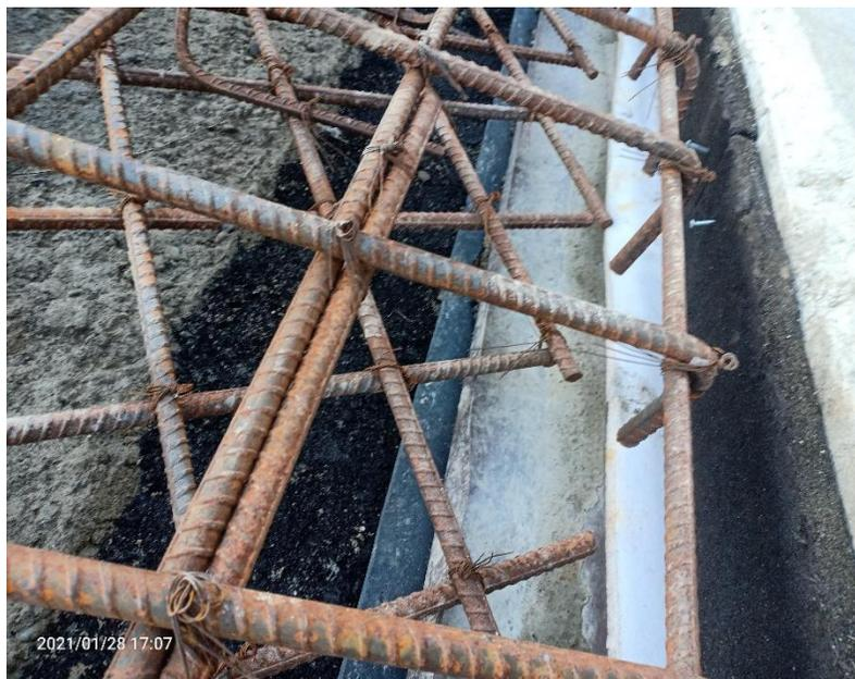
Fig: Details of perimeter joint (Sand asphalt mixture, Hypalon band, Copper water stopper, Polyurethane foam and Bitumious fiber from bottom to top).
