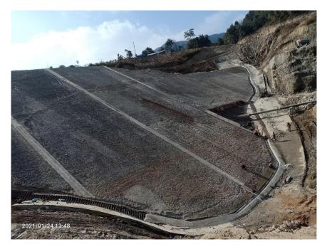
Fig. Zigzag line of perimeter joint due to undulated and curved profile of plinth at Dhap Dam.
