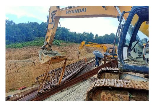
Fig: Loading Slipform on rail for trial running
