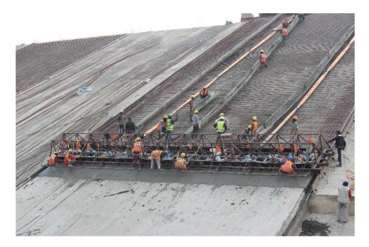
Fig: Concreting on S-5 panel with slipform using double winch, adding extra dead load, joining platform for labour to sit while trowling.
