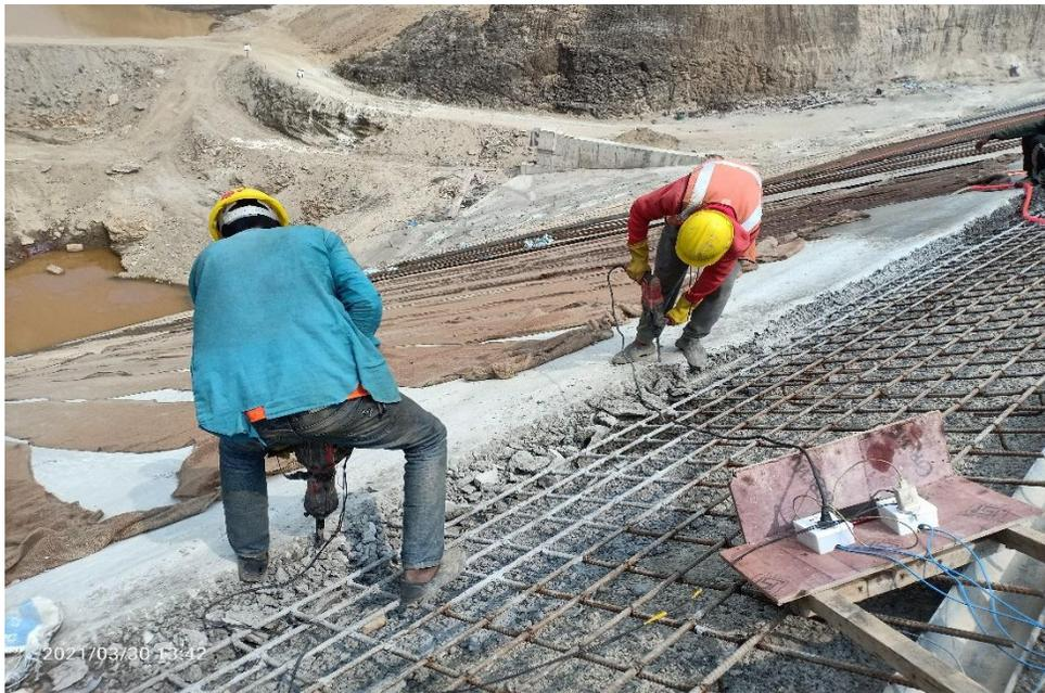
Fig: Removing loose concrete from joint using jack hammer
