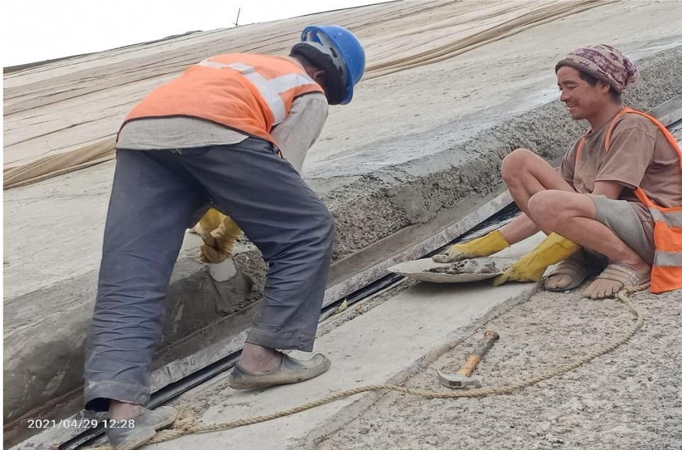
Fig: Repairing honeycomb concrete with repairing mortar
