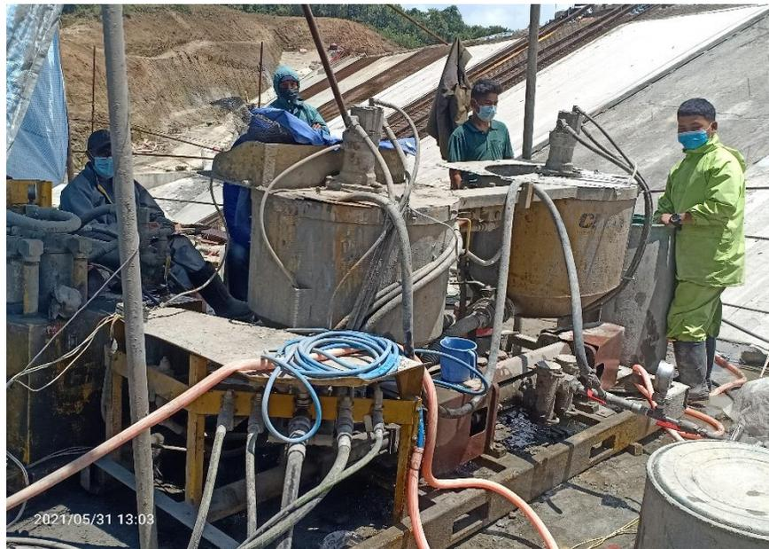
Fig: Colloidal mixture, agitator, piston type grout pump, digital flowmeter set
