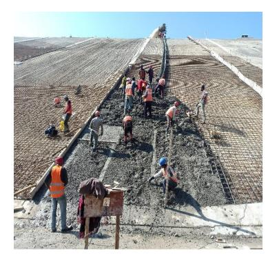
Fig: Starter slab concreting
