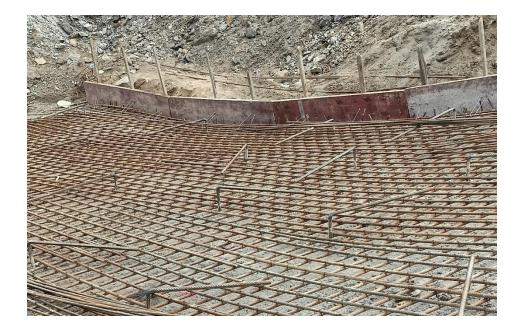
Fig. Plinth reinforcement and Anchor bars at external plinth
