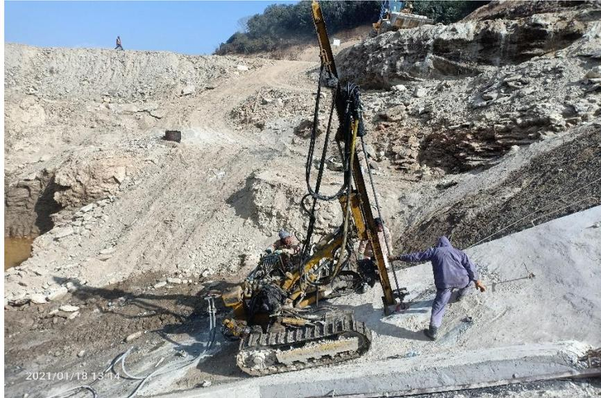
Fig: Normal drilling with ROC machine
