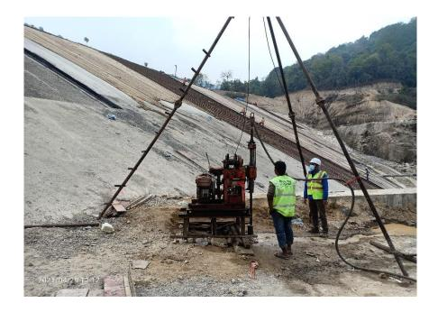
Fig: Rotary drilling machine for core drilling
