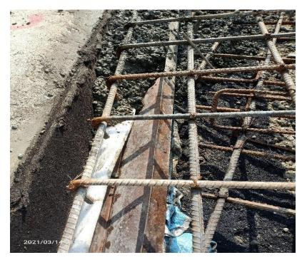
Fig: Polyurethene foam pressed down by fresh concrete of starter face slab
