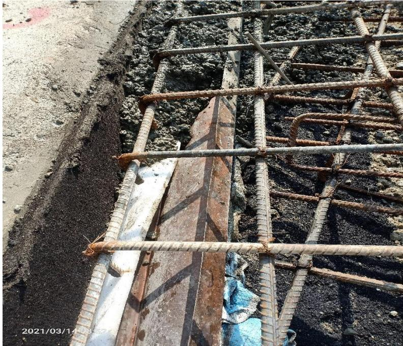
Fig: Polyurethane foam pressed down by fresh concrete of starter face slab
