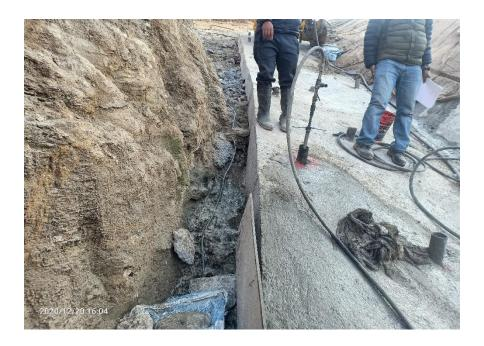
Fig: Side leakages of grouting
