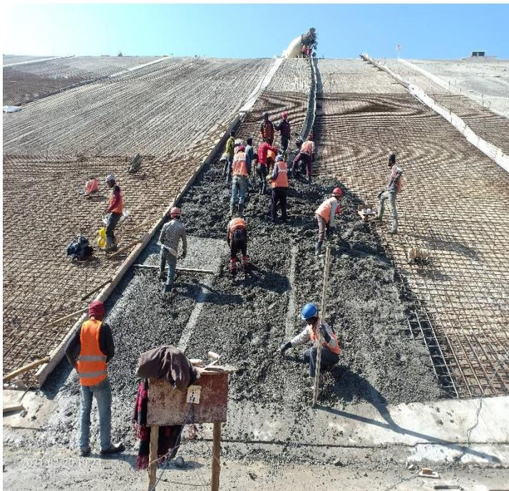
Fig: Starter slab concreting
