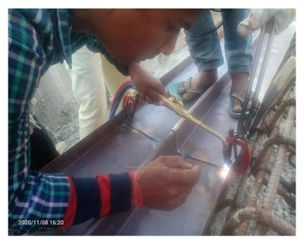
Fig: Brazing of copper water stopper.
