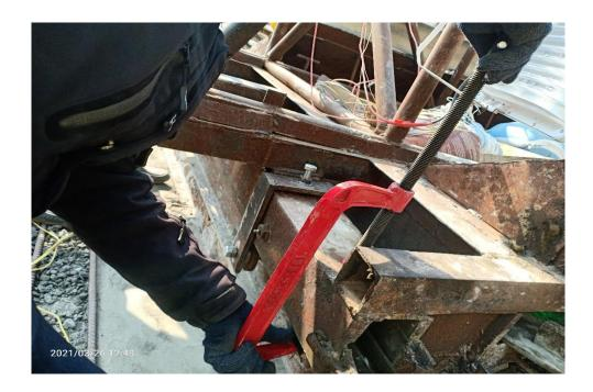
Fig: Clamping the slipform with rail
