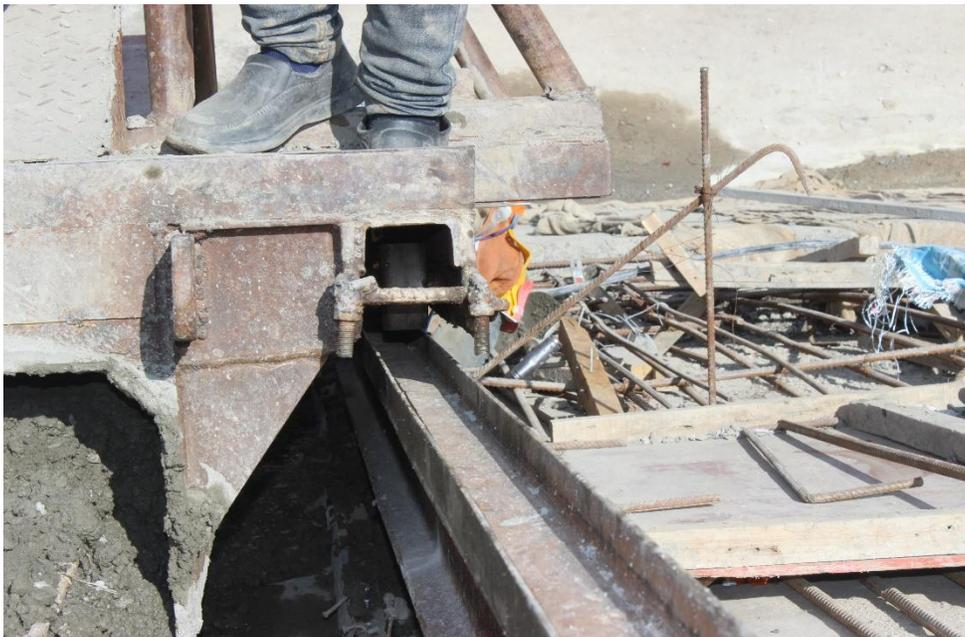
Fig: Uplifting of slipform guide roller on S-9 panel during concreting
