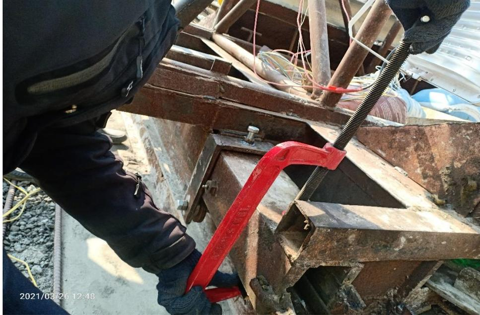
Fig: Clamping the slipform with rail
