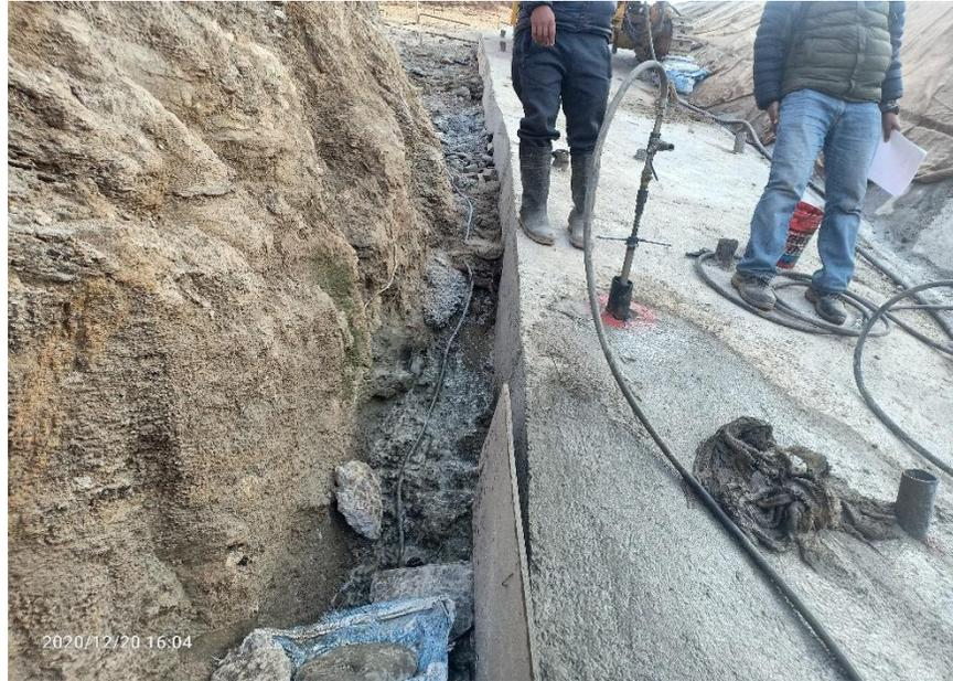
Fig: Side leakages of grouting
