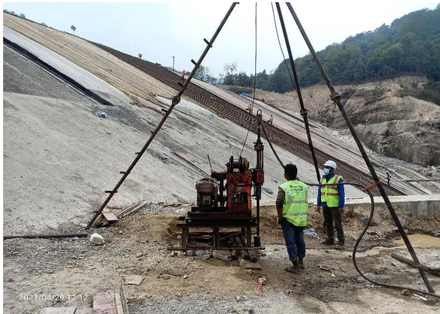
Fig: Rotary drilling machine for core drilling
