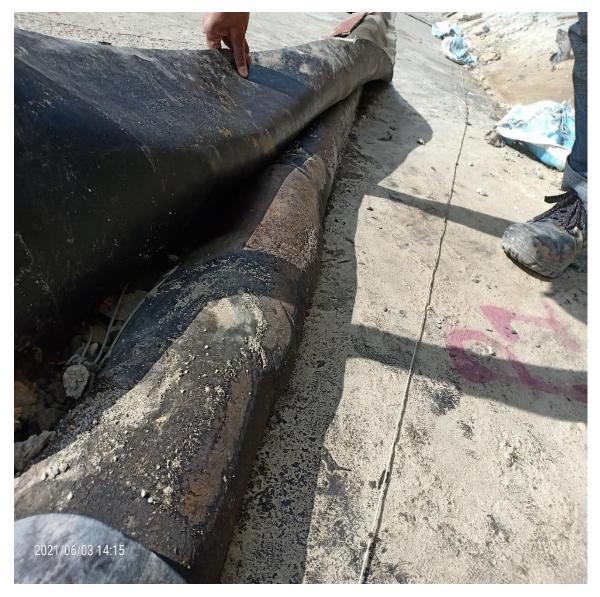
Fig: Disfigured shape and some minor head cracks on the surface of mastic mound due to lack of proper covering
