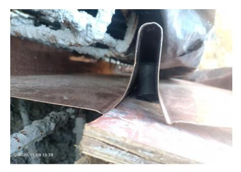
Fig: Neoprene not filling the full depth of rib of copper water stopper
