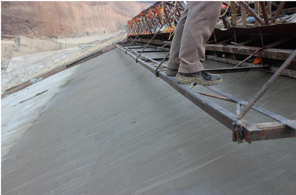
Fig: Finished surface of face slab
