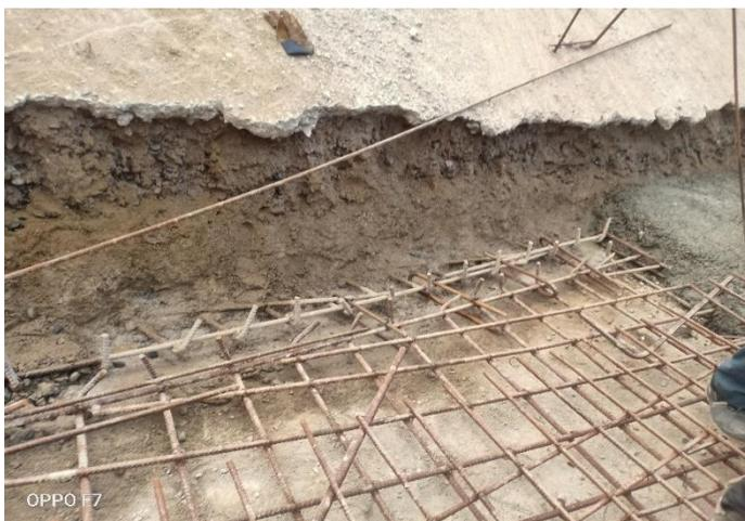
Fig. U reinforcement bar tied between internal and external plinth.
