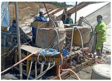
Fig: Colloidal mixture, agitator, piston type grout pump, digital flowmeter set
