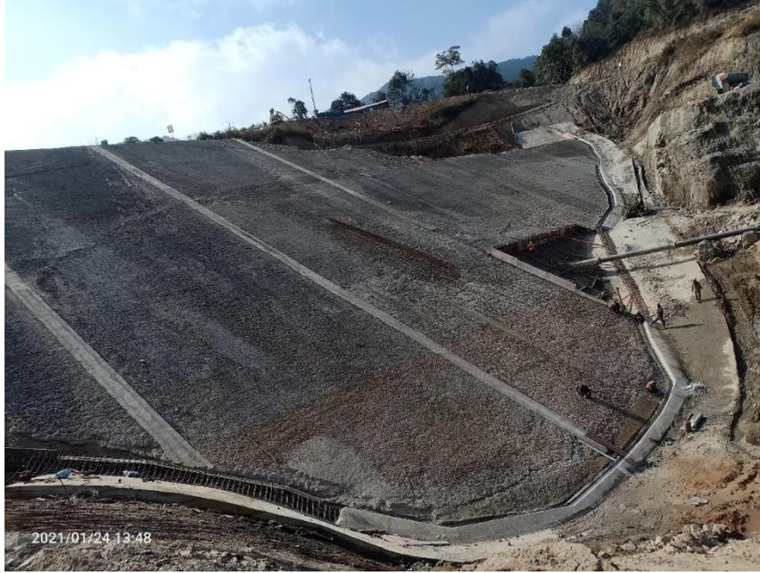
Fig. Zigzag line of perimeter joint due to undulated and curved profile of plinth at Dhap Dam.
