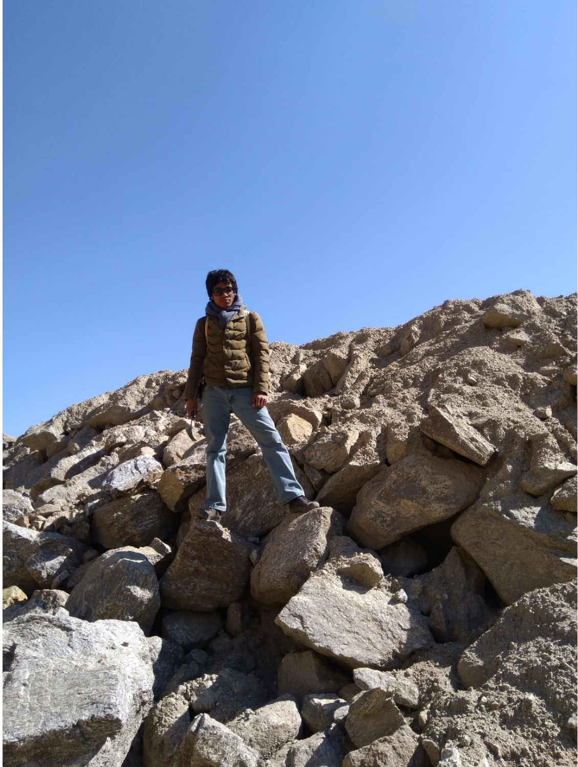
Plate 8: Rock boulders for the embankment construction
