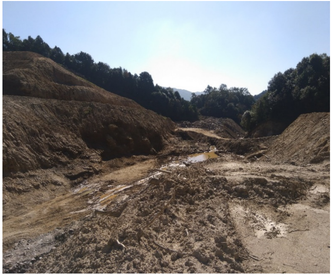
Plate 2: Downstream section of the study area, from the right bank
